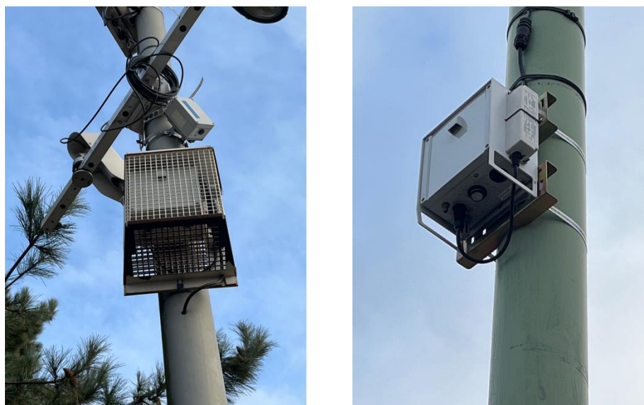
Figure 4: Aeroqual AQY1 units, as supplied by Telensa (left) with additional housing and CIMCON (right) mounted directly.
