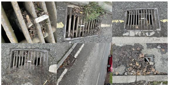
Figure 49: Photos of sensors showing accumulated debris on the sensor installation (photos: H Steventon)
