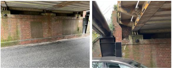
Figure 22: Sensors installed on Coddenham Road Bridge (photographs: H Steventon) Image on the left shows CRB2 on the left, CRB1 on the right Image on the right shows potential for car to trigger distance measurement
