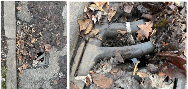
Figure 27: Nowton Road Gully 1, as initially located, and after minor leaf clearance to reveal sensor (Photo: H Steventon)
