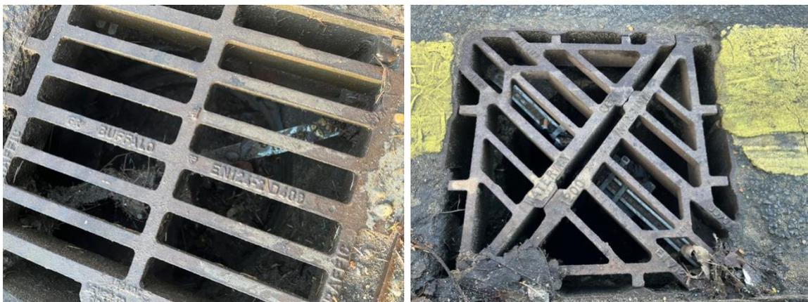
Figure 51: InTouch sensors installed with bar diagonally across gully anticipated to cause problems with gully cleansing.
