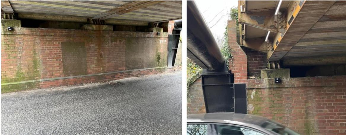
Figure 22: Sensors installed on Coddendam Road Bridge (photographs: H Steventon)
