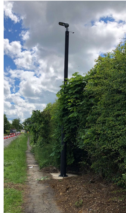
Installation of solar PV columns with integrated batteries on pathway
