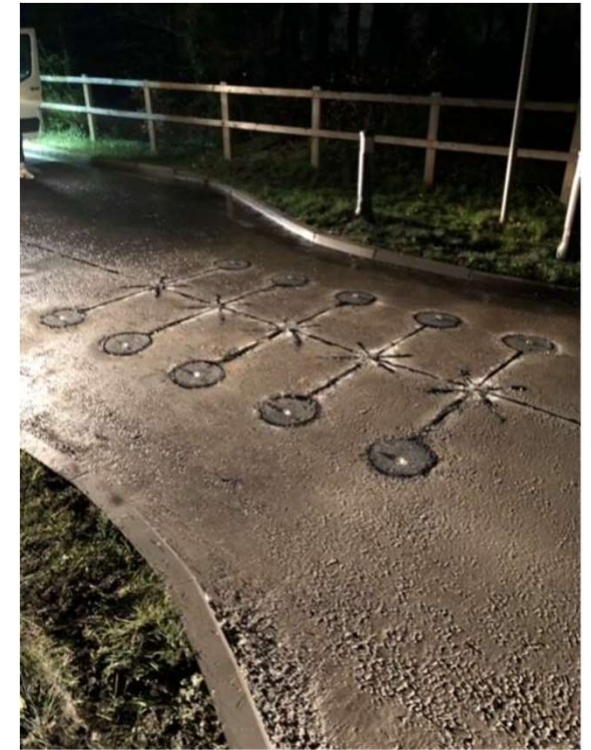
Installation of kinetic road prototype units on access road to household waste recycling site
