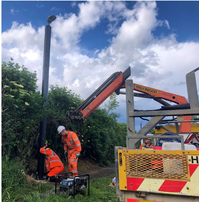
Installation of solar PV columns with integrated batteries on pathway
