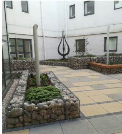
Basildon Hospital Rain Garden (SuDS)
