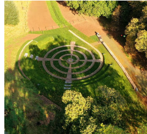
Sidmouth flood alleviation scheme
