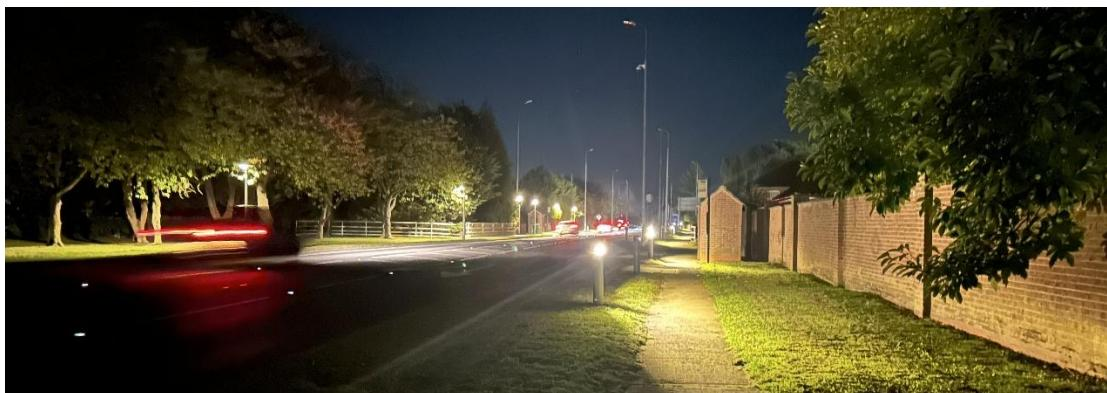
**Hayton Village** – Low Level pedestrian Lighting, Solar Studs and High Reflectivity Lines replacing Street lights
