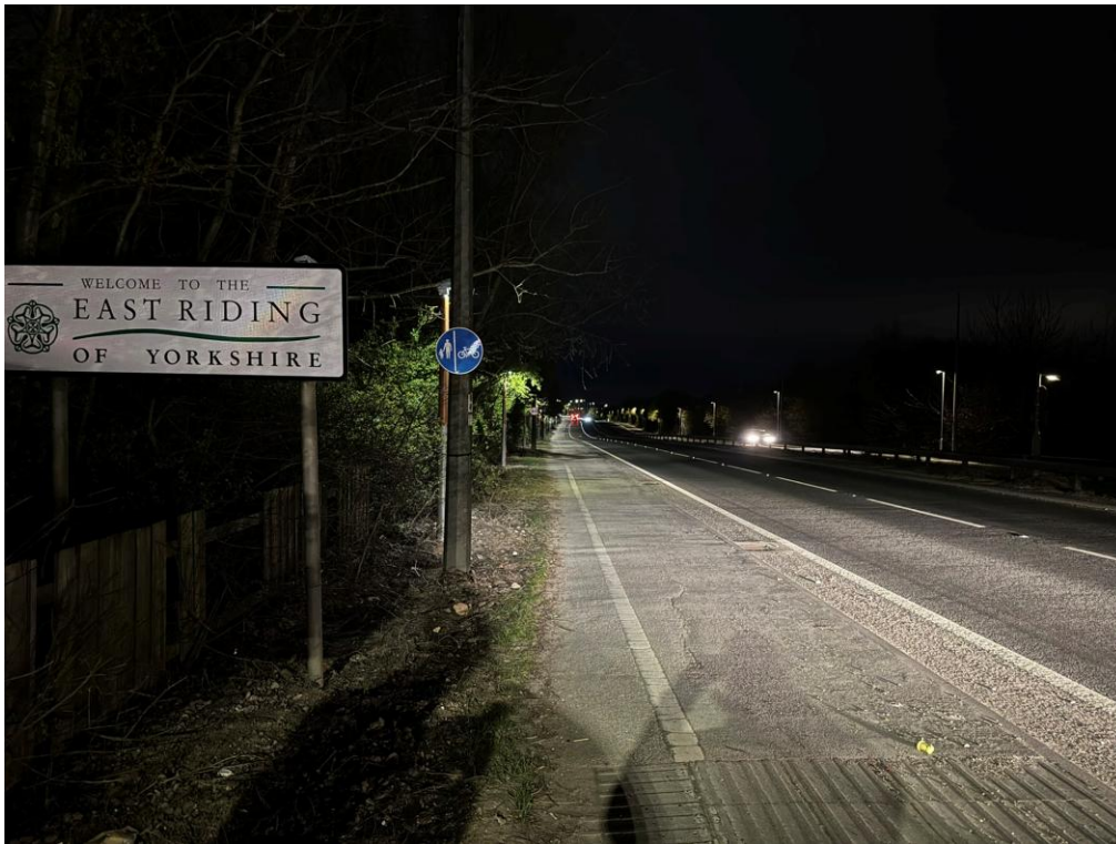
[Pedestrian Lighting A1079 Raich Carter Way]
