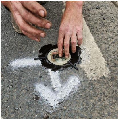
[Installation of illuminated road stud / Installation of road markings / Category 3 sign]
