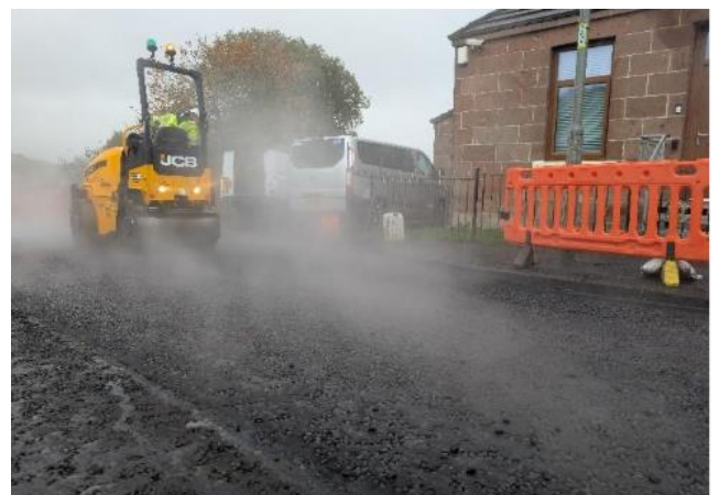
Figure 2: Flattening process of the material
