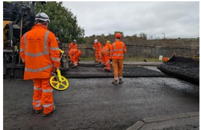
Figure 1: Laydown of the EcoFlakes
