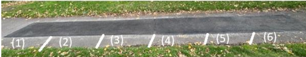
Figure 4. Trial 1, Walkway surface conditions
