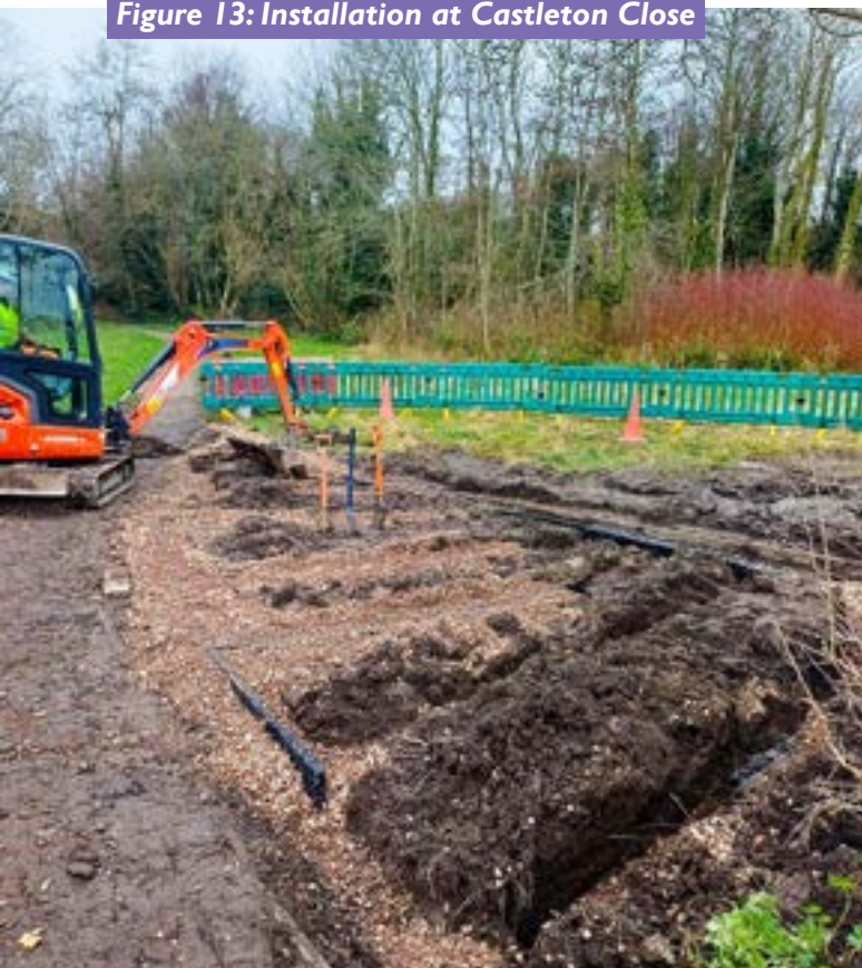
Figure 13: Installation at Castleton Close
