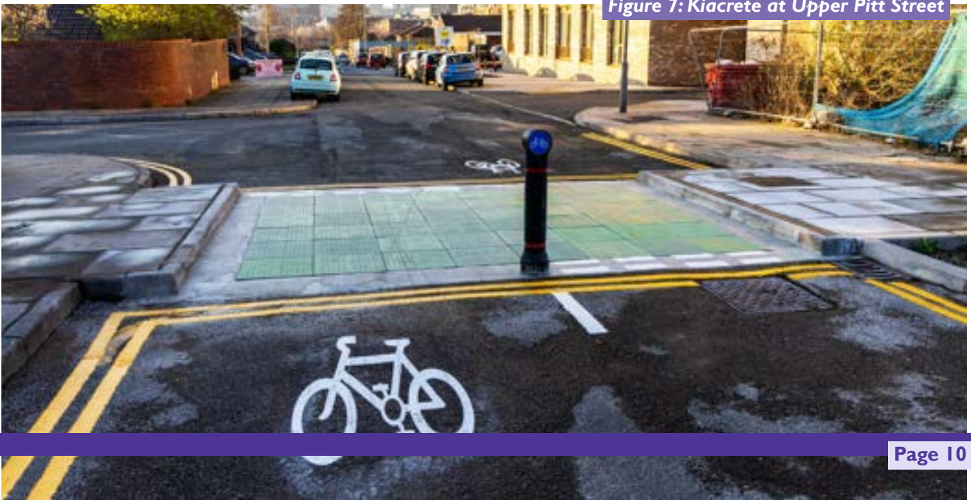
Figure 7: Kiacrete at Upper Pitt Street
