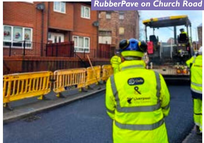
Figure 9: Installation of RubberPave on Church Road
