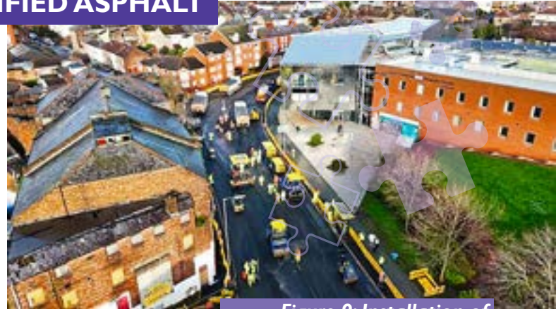
Figure 9: Installation of RubberPave on Church Road
