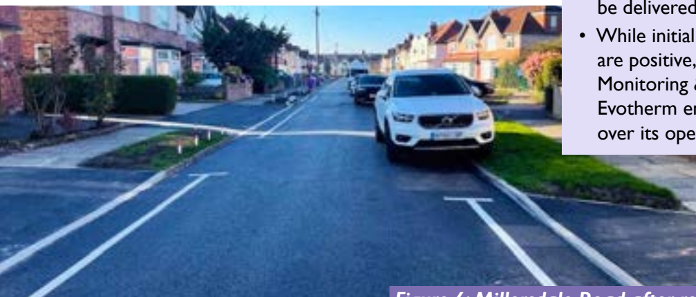
Figure 6: Millersdale Road after resurfacing
