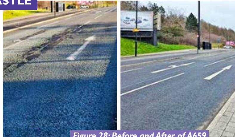
Figure 28: Before and After of A659 Scotswood Road, Newcastle
