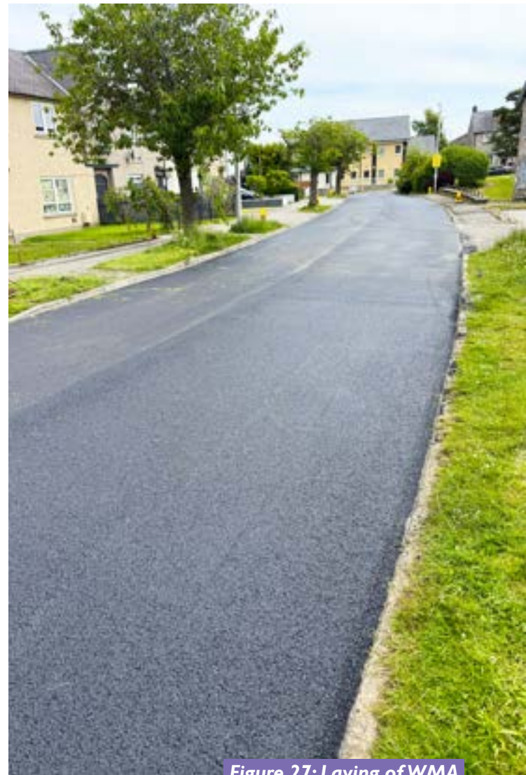
Figure 27: Laying of WMA SMA at Byron Crescent
