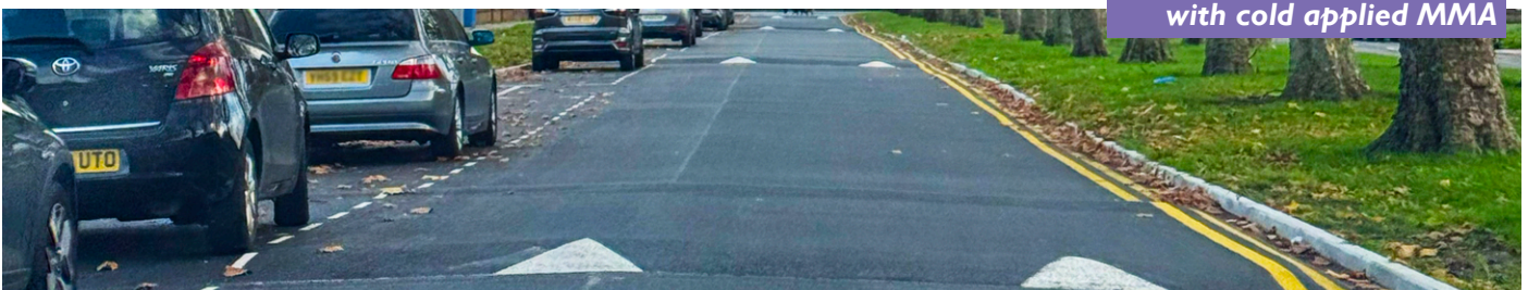
Figure 14: Pinehurst Avenue with cold applied MMA
