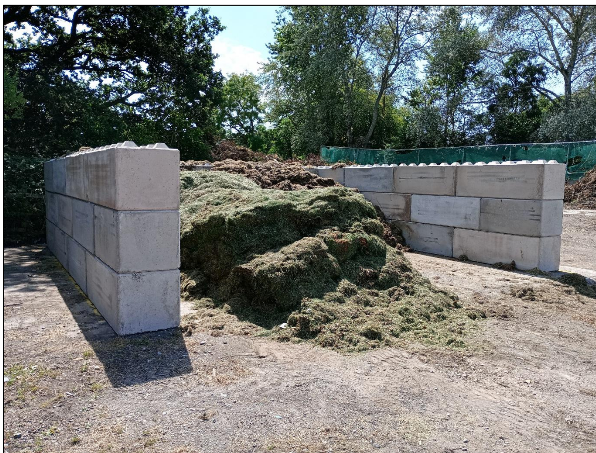
Concrete block grass storage bay – South Gloucestershire Council depot, Broad Lane, Yate.
