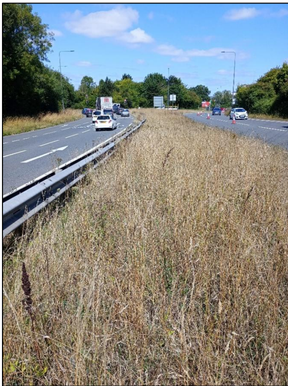
Site 1 – (A4174) before cutting
