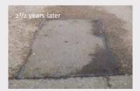
The images on the left show the complete patch repair applied to a defect. Over a  $2^{1/2}$  year period, this patch repair has not required any follow-up maintenance – as shown in the bottom image.
