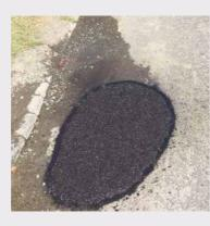
management, where extremely low temperatures exist or where there is standing water. The Council has found that the one consistent item in the process is the use of overbanding to protect the newly formed joints.
